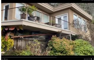
In early 2022 a house in the Magnolia area of Seattle slipped off it's foundation during a record rain storm. It is located on Perkins lane which has previously been the site of several homes that have been destroyed on the hill.
